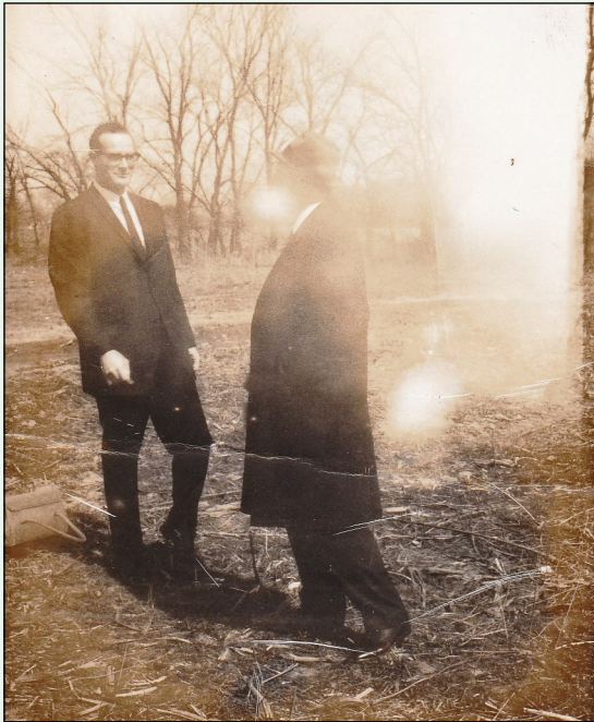
It's been 60 years since the Fairfield Municipal Building opened for business. This photo from the Fairfield Echo archives shows Council President Glenn Maddox (left) with Fairfield Mayor Edwin Bartels at the groundbreaking .
